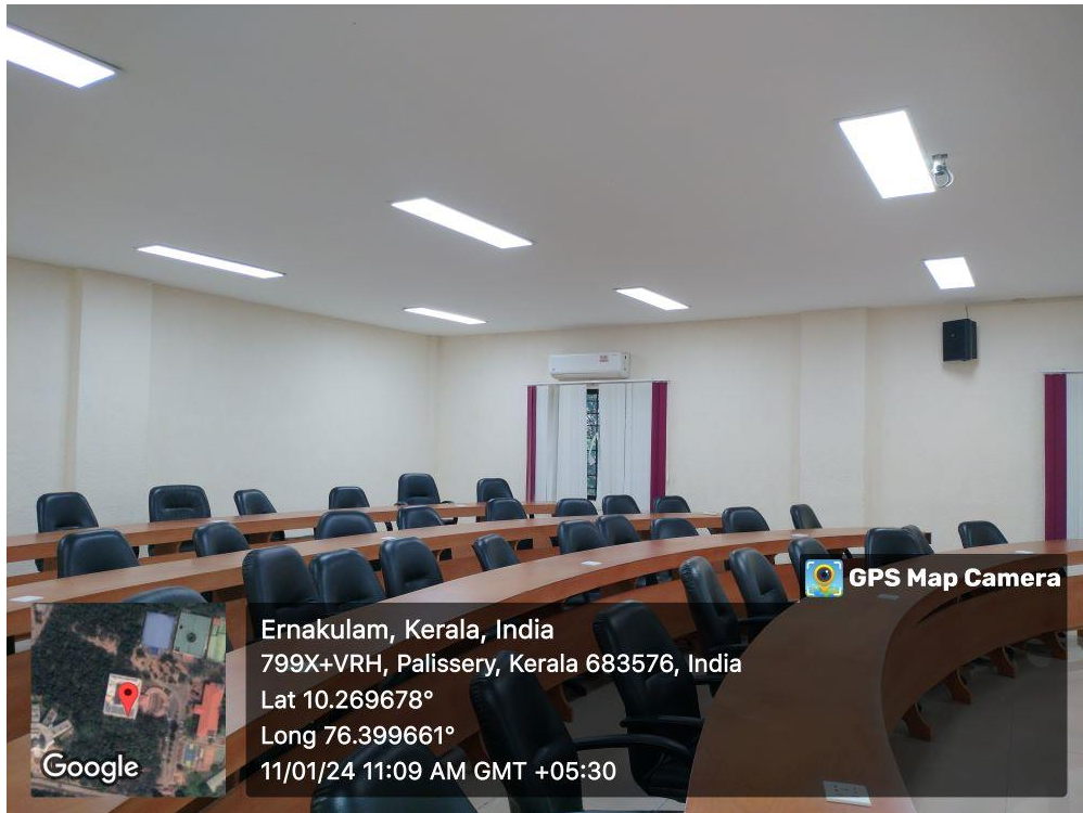
LED lights installed in Conference room at Administrative Block
