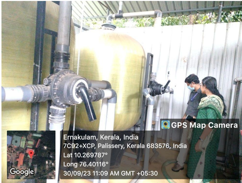
Water treatment Plant being inspected
